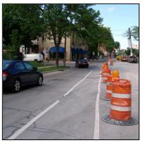
Bicycle lanes and access should be maintained through street construction or projects that impede into the bike lane.
